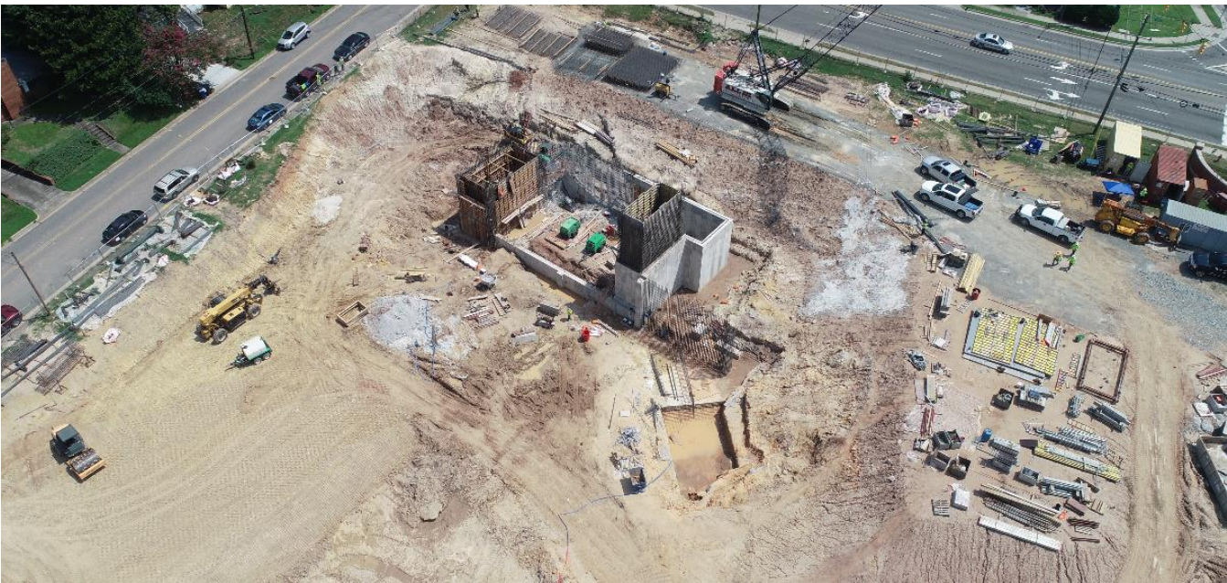
New School of Business – Aerial View – August - 2021.
